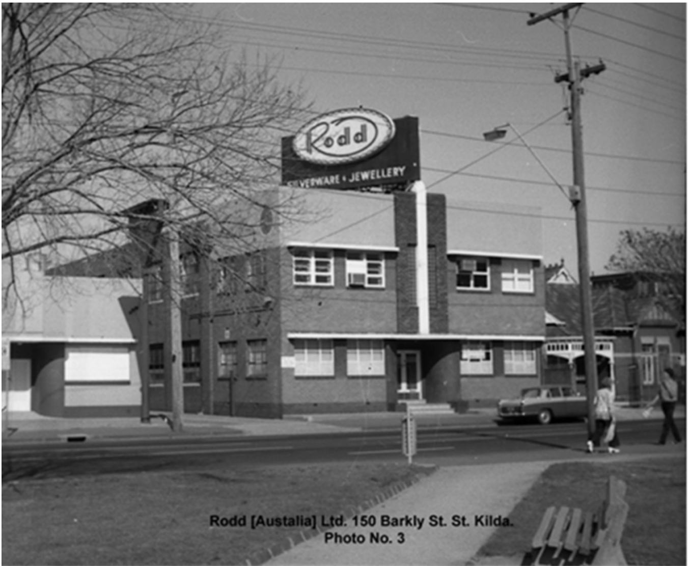
1A, 1B, 1C: This brick building had two floors. The top floor consisted of the executive offices (1A), the administration office (1B), and the knife assembly and finishing department (1C). The total lower floor was in three sections, the finished goods warehouse and managers' office at the Barkly Street end. The Greeves Street end was the dispatch department. Photograph courtesy the Bruce McCullough Collection.
